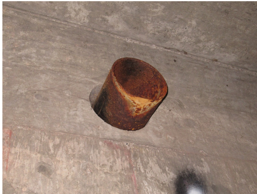
Photo 14: 8" Metal Drain Pipe Corrosion
