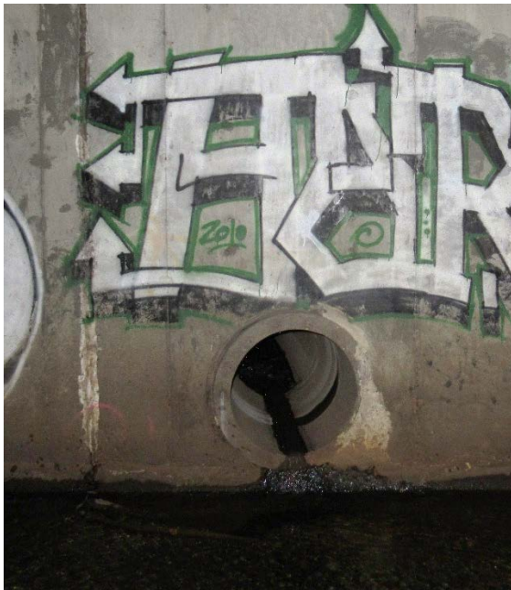
Photos 11/12: 24" RCP Storm Inlet - segment 17, north wall
