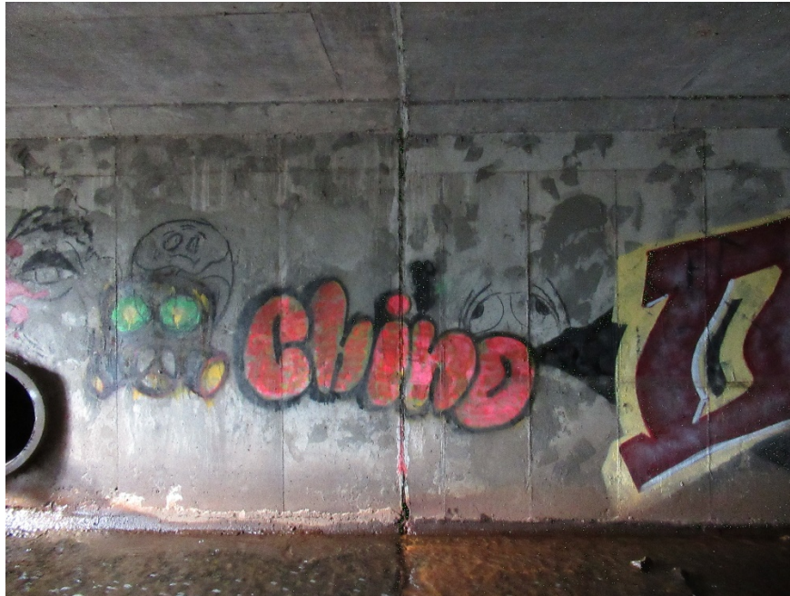
Photo 6: Typical Joint between Box Culvert Segments joint 2 (north) pictured
