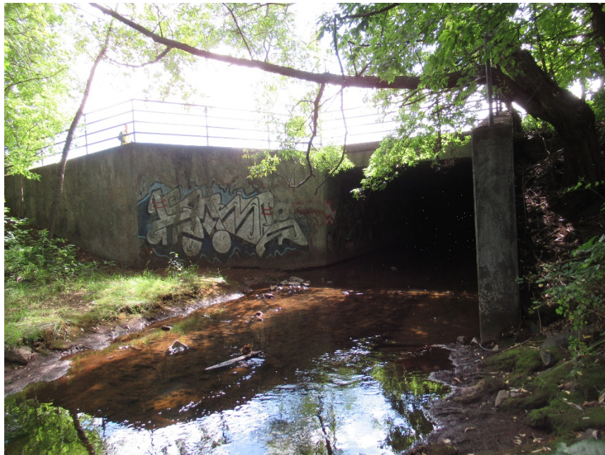
Photo 20: Outlet Headwall and Wingwalls
