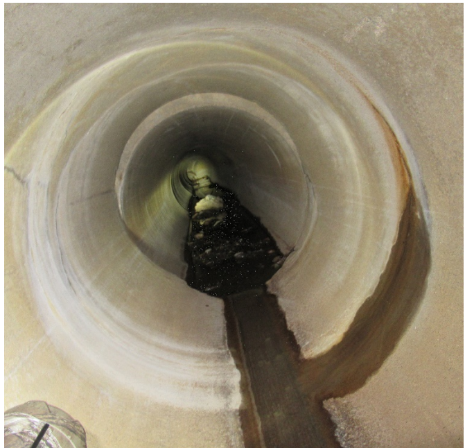
Photos 11/12: 24" RCP Storm Inlet - segment 17, north wall
