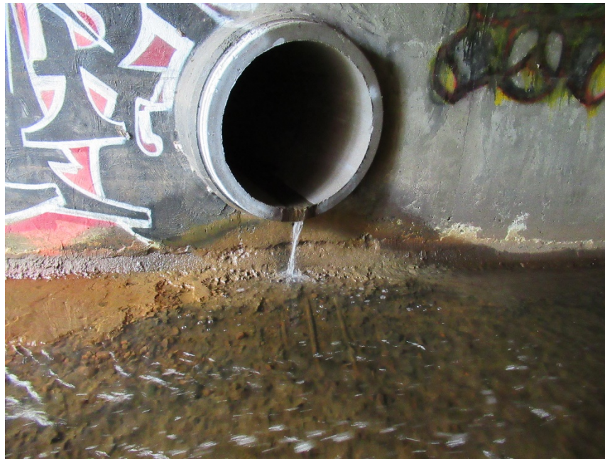
Photo 5: Deep Scour in Floor at RCP Outlet near Inlet of Culvert note exposed reinforcing in floor
