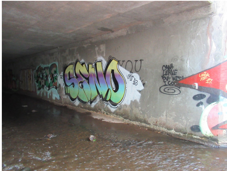
Photo 4: Culvert Floor Typical Condition note scour through middle & intact floor at edge
