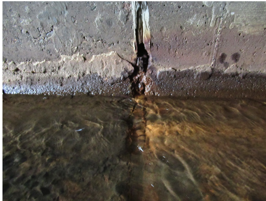
Photo 8: Typical Deteriorated Floor Joint joint 2 pictured
