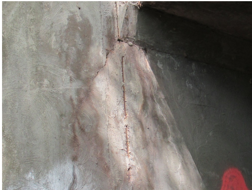
Photo 2: Culvert Section 1 (inlet, north wall) Exposed and Corroding Reinforcement also note crack in wingwall with rust staining
