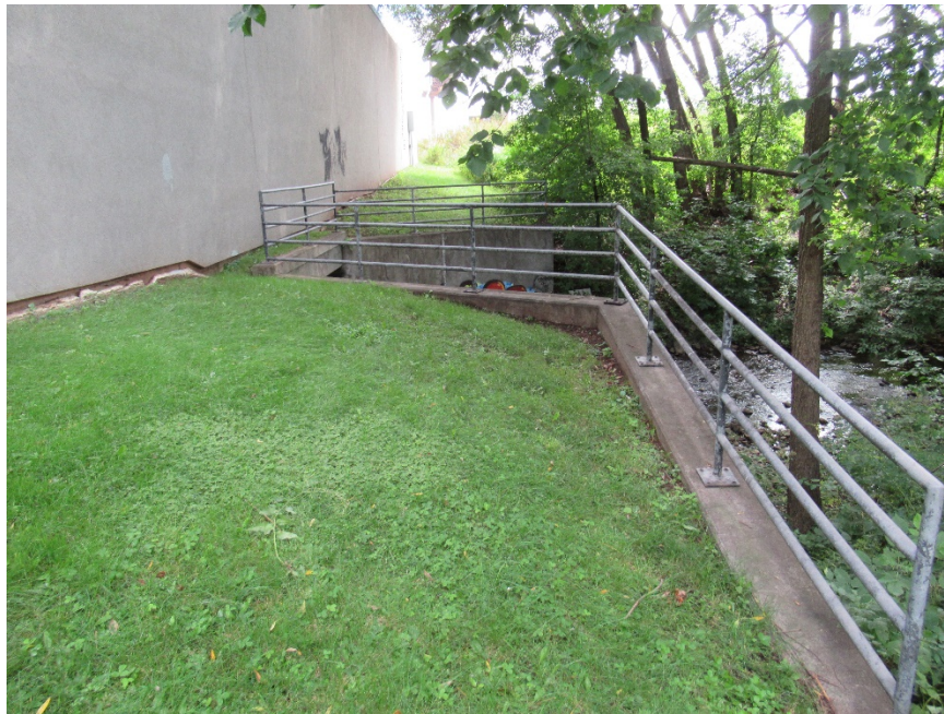
Photo 17: Inlet Headwall/Wingwall Metal Railing
