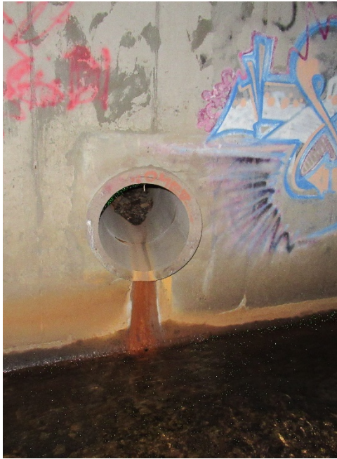
Photos 9/10: 18" RCP Storm Inlet - segment 15, south wall
