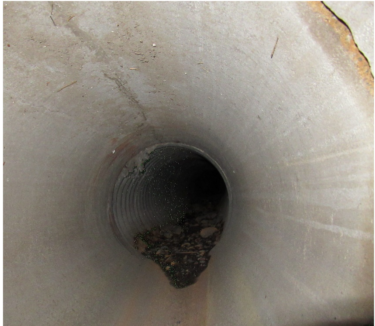
Photos 9/10: 18" RCP Storm Inlet - segment 15, south wall
