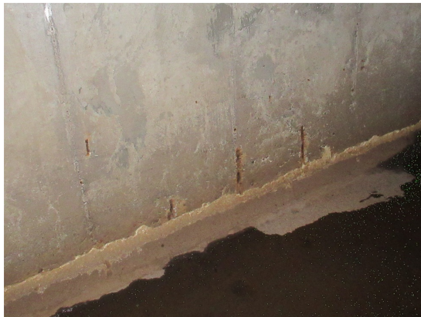
Photo 3: Culvert Section 6 (north wall) Exposed and Corroding Reinforcement
