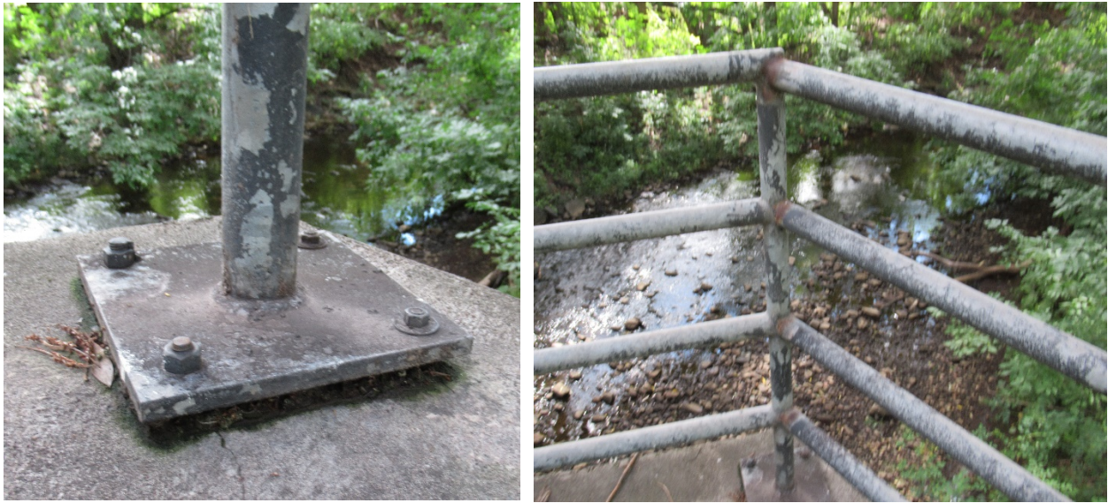
Photo 18/19: Railing Base Plate & Coating Condition
