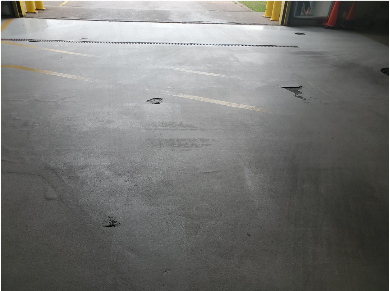
Main Bus Entry, spalled concrete, recoating
