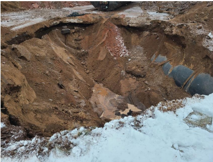
Excavation after removal of two tanks. Groundwater visible in tank basin, along with remaining tank.
