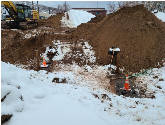
View of second and third tanks in tank basin during removal.
