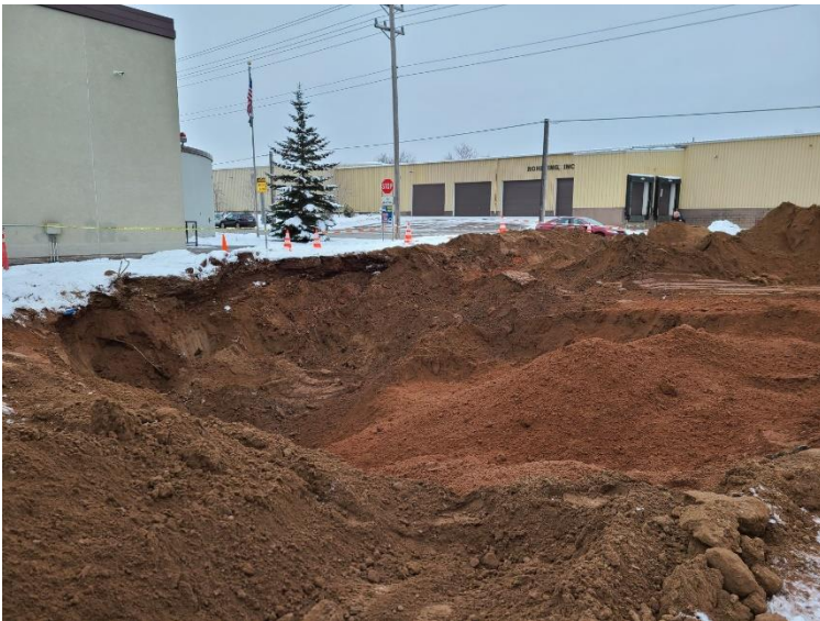
Excavation being backfilled following tank removals.
